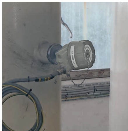
COMPACT SENSOR FOR BROKEN BAG DETECTION
