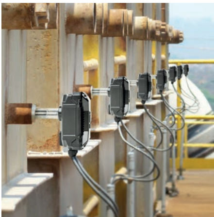
BROKEN BAG DETECTION WITH EXTERNAL DISPLAY
